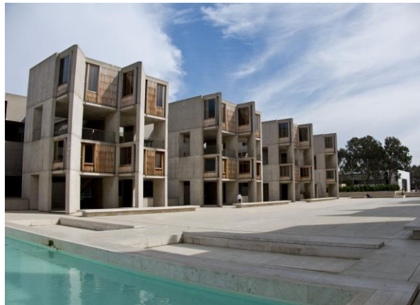
Salk Biological Institute, North Wing Towers. © Getty Conservation Institute.
