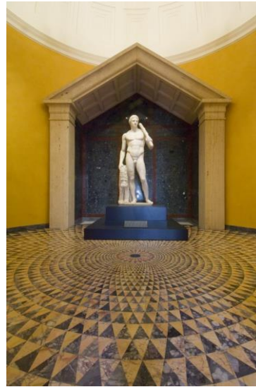
6. Temple of Herakles gallery, with alternating triangles of Numidian yellow and africano or dark gray Lucullan marble, at the Getty Villa Photo: Richard Ross © 2005 Richard Ross with the courtesy of the J. Paul Getty Trust
