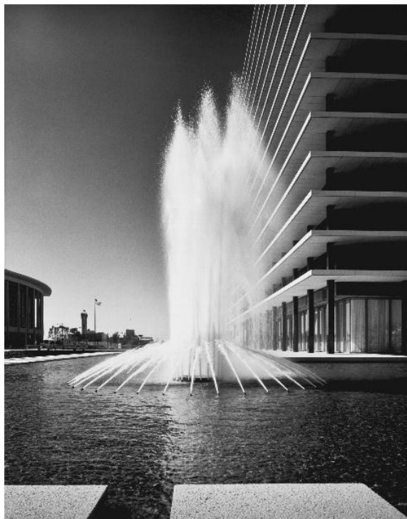
Department of Water and Power Building Corner with Fountains, 1965. Photo: Julius Shulman (American, 1910–2009). Gelatin silver print. The Getty Research Institute, Los Angeles. © J. Paul Getty Trust
